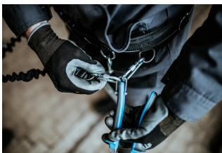
The carabiner on the lanyard has to be protected against opening using a lock ring.
